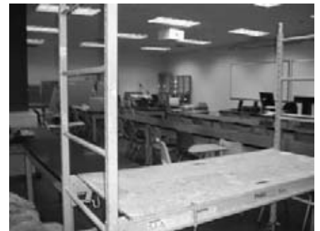
New classroom, under construction, late summer.
