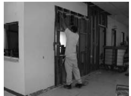
New Department Office under construction, late summer.
